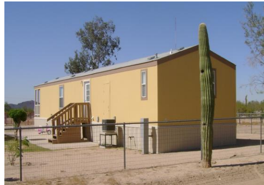
Elevated Mobile home with elevated utilities
