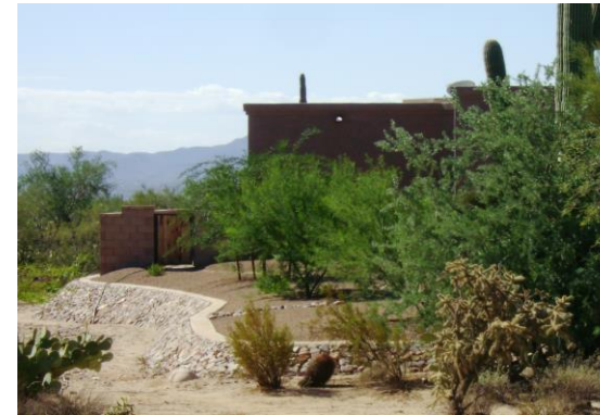
Elevated Home with riprap scours protection
