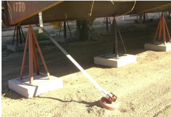
Anchor and support system for Mobile home
